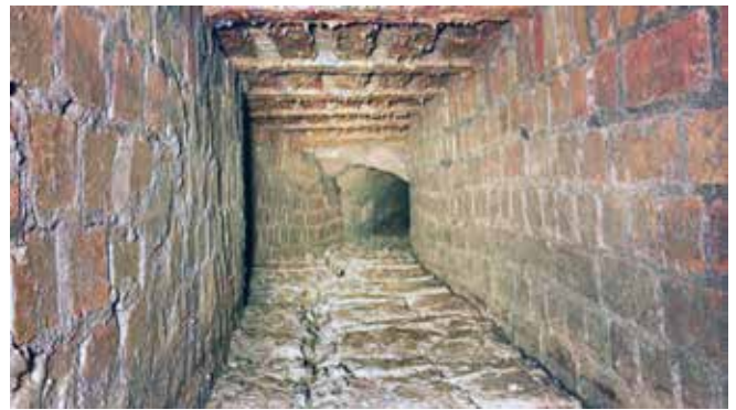
Church Aston culvert
